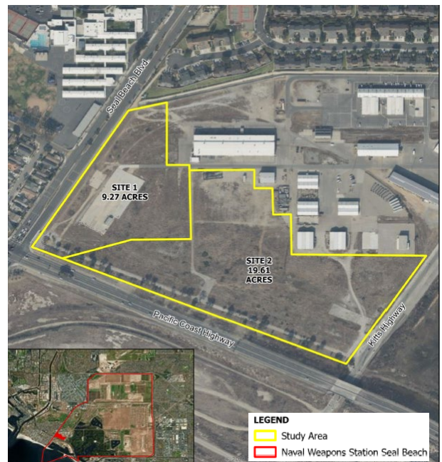
Aerial view of the proposed Site 1 and Site 2 from NWSSB, looking south.
